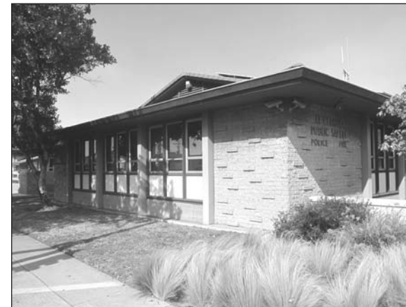
El Cerrito’s Public Safety building
